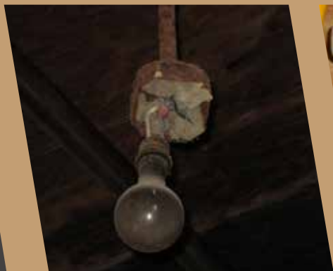
Corroded light fixture and electric plug demonstrate the corrosive nature of dry fertilizers; the mislabeled bin of red potash can lead to application errors.
